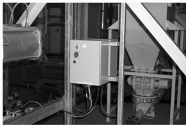
Figure 1.14: Old solution: Motor control - panel mounted decentrally
